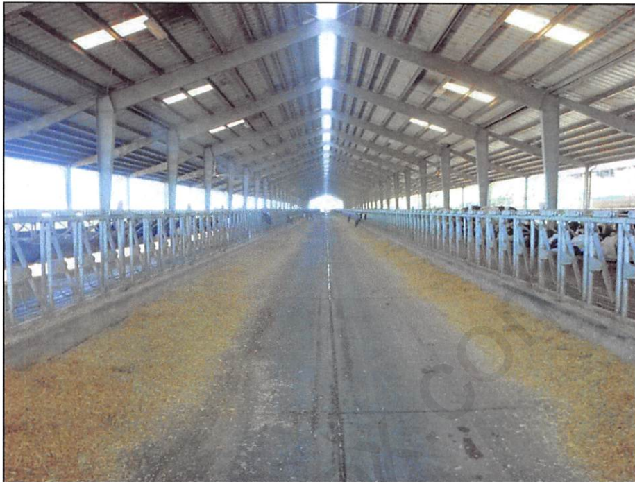
Photograph 5. View down the central feeding alley of the lower 1,000-cow freestall barn. Photo by A. D'Angelo; 12/14/16.
