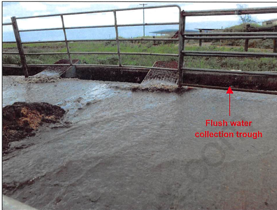
Photograph 13. Flush water from the 380-head calf barn is captured in a collection trough located at the end of the barn and conveyed to the manure composting building collection pit, shown in Photographs 15 and 16. Photo by A. D'Angelo; 12/14/16.
