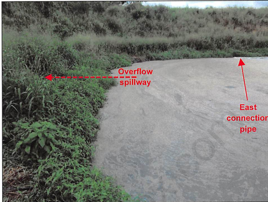
Photograph 31. View, facing south, of the approximate location of the lower lagoon overflow spillway. Photo by A. D'Angelo; 12/14/16.
