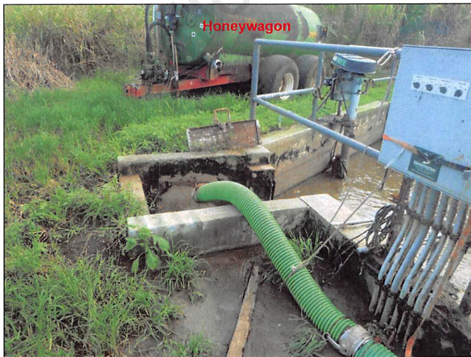
Photograph 20. View of the manure composting building collection pit overflow point. Overflow flows into the manure separation cells shown in Photographs 22 and 23. Note the honeywagon. Photo by A. D'Angelo; 12/14/16.
