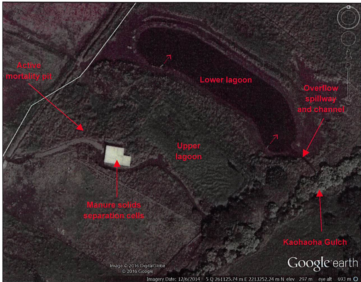
Figure 2. GoogleEarth aerial image of the BID manure separation cells and wastewater lagoons, imagery date December 6, 2014. The red arrows and callouts are approximate location estimations of Facility features observed during the inspection, described in the report, and shown in the Photograph Log.
