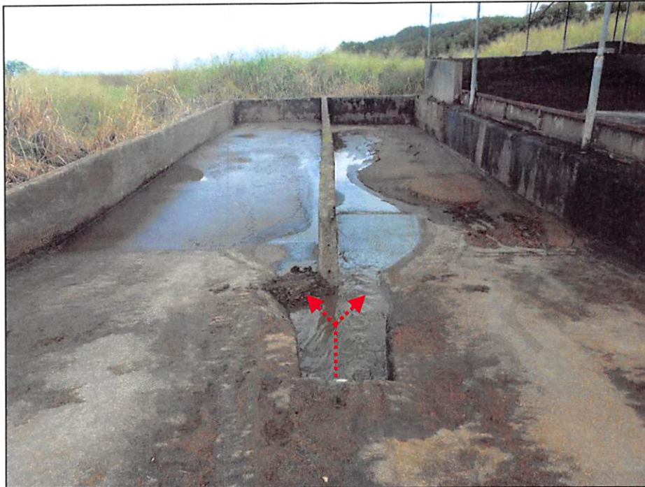
Photograph 23. View of flow from the manure composting collection pit entering the primary cells of the manure solids separation cells shown in Photograph 22. Photo by A. D'Angelo; 12/14/16.
