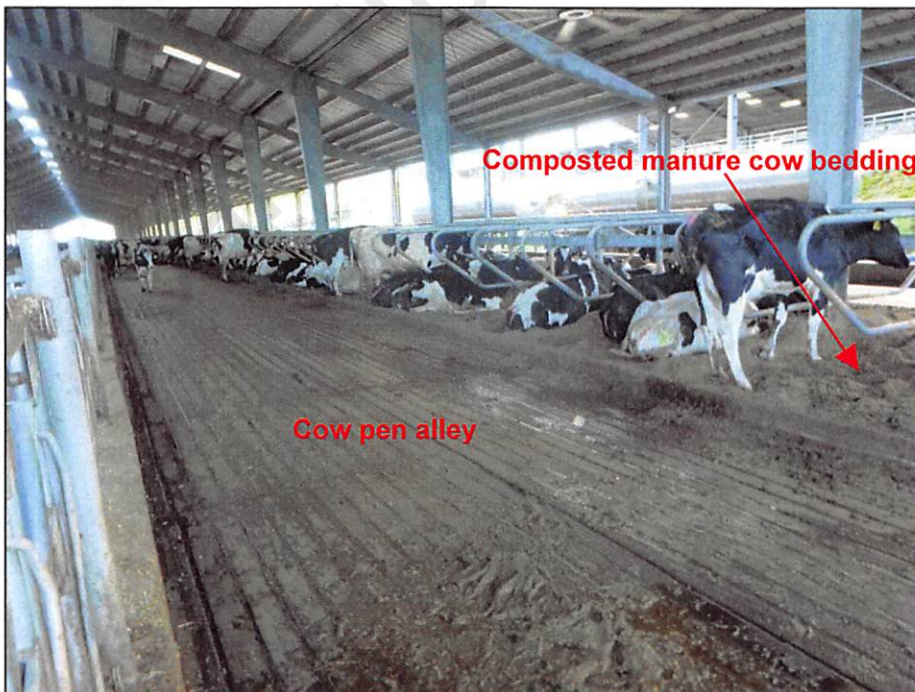
Photograph 6. The cow pen alleys of the freestall barns contain mechanically operated manure scraping systems that scraped manure toward and into a collection trough in the center of each barn. The cow pens were lined with composted manure bedding that is made onsite using recovered manure solids. Photo by A. D'Angelo; 12/14/16.
